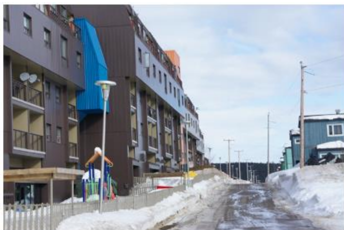
The 1.3 kilometre-long climate wall shelters the residential district of Fermont. Photo: P. Hemmersam.
